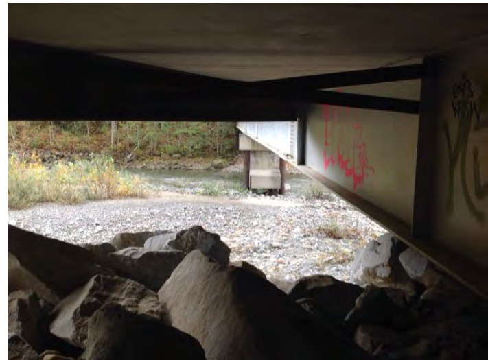
right bank upstream girder flare
