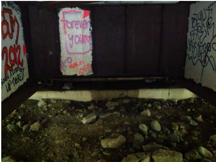
right bank main span girder bearing
