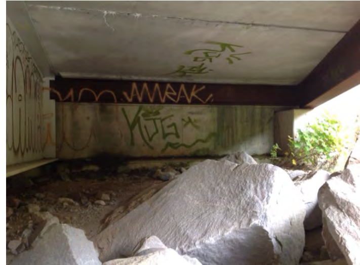
right bank upstream girder flare
