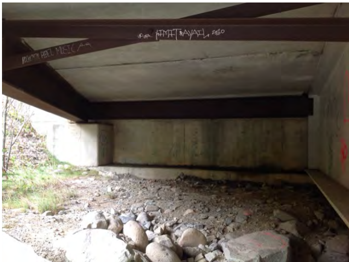
right bank downstream girder flare
