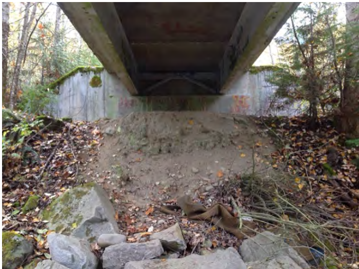
Left Bank Abutment when facing downstream
