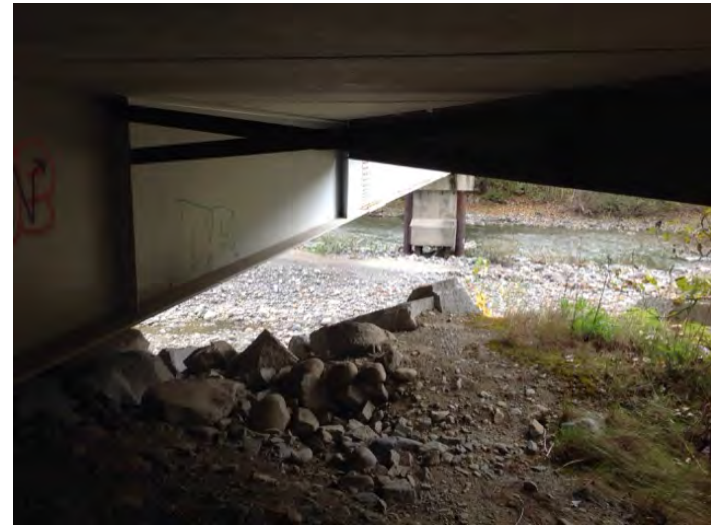
right bank downstream girder flare
