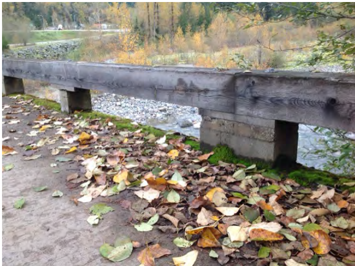
Guardrail on span 2
