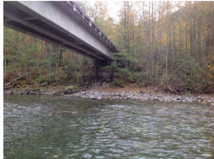
pier 1 and left abutment
