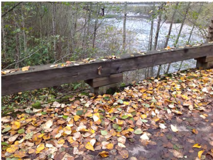
Guard Rail on span 1
