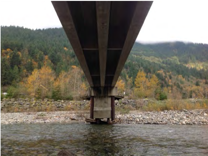
span 2 superstructure, pier 2
