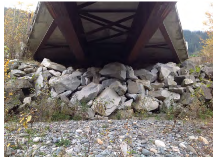
Right Bank Abutment when facing downstream
