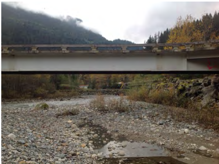
span 3 splice plates
